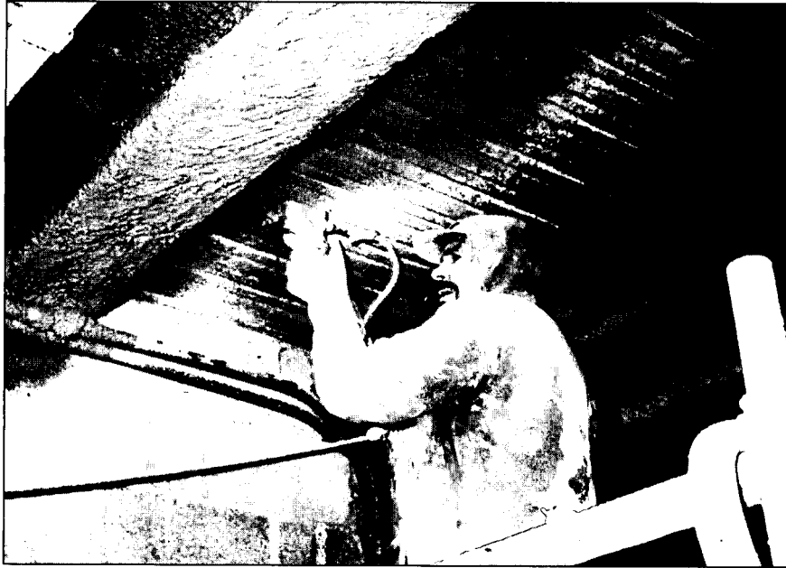
Figure 7.9 Sprayed fire protection
